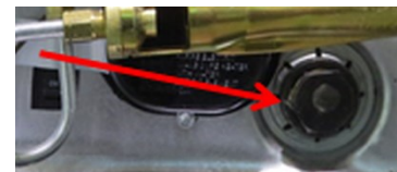
Typical anode rod, installed
