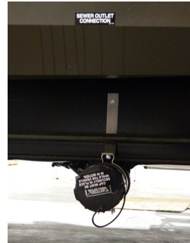
Sewer outlet connection, located on the off-door side under the kitchen slide.
