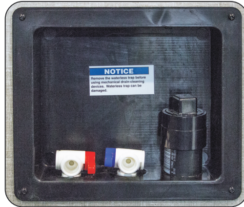
Hot & Cold Water Washer Hookups
