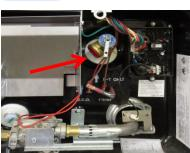
The arrow in the above photo shows the P&T relief valve location on this particular water heater model.
