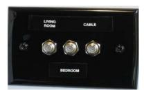
Typical exterior cable and satellite connection plate, located in the utility center.
