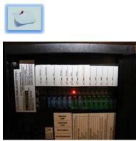
A red light (as shown in the above photo), typically indicates a blown or missing fuse in the load center.
