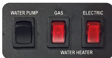
Water Pump & Water Heater On/Off Switches
