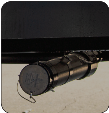
Sewer Outlet Connection Is Located Under the RV on the Off-Door Side
