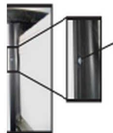
Step 1 – Typical Schwintek motor retention screw location, viewed from inside the RV.
