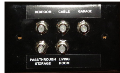
Typical cable/satellite outlet, located in the utility center
