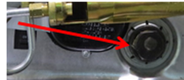
Typical anode rod, installed
